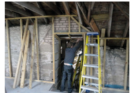
Framing out the upstairs lounge
