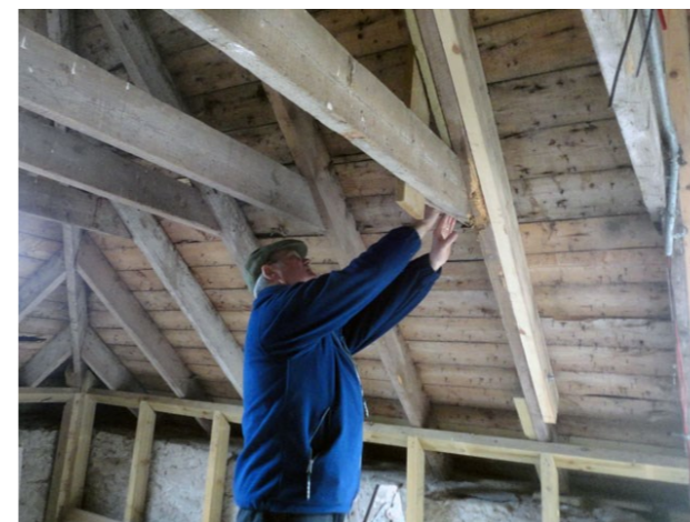
Tom makes sure that this new beam is now secure
